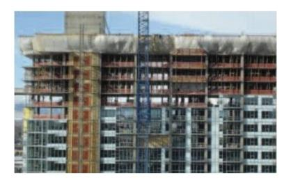
The high-rise contains two massive concrete cores with walls up to three-feet thick which were created using approximately 8,000 cubic yards of SCC and a new stateof-the-art admixture technology, ADVA®408.
