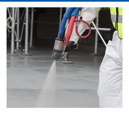
The airport construction in Ireland required below ground waterproofing of the basement area, specifically the walls as well as reinforced concrete columns. Situated on a sloping site, the engineers designed below grade drainage under the slab, as it was not a monolithic basement. Therefore, a membrane suitable for application in damp areas was also called for.
