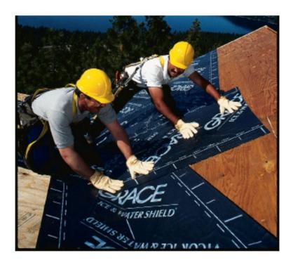
Consistent with good roofing practice, install the membrane such that all laps shed water. Always work from the low point to the high point of the roof. Apply the membrane in valleys before the membrane is applied to the eaves. Following placement along the eaves, continue application of the membrane up the roof. The membrane may be installed either vertically or horizontally.
